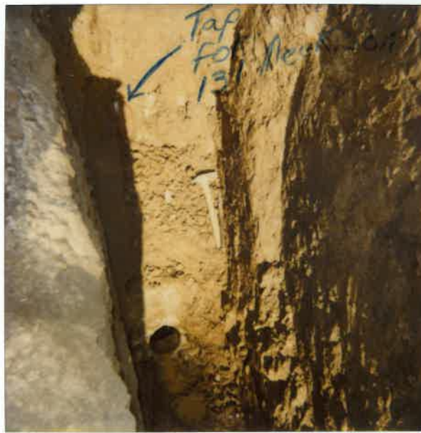
203 Meekison 21" Brick Mun 8-22-91 8'8" F/L Top of Pavement
